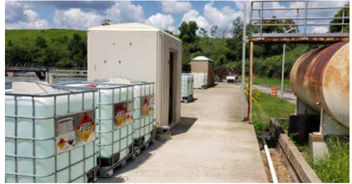
Parsippany Troy Hills Township Wastewater Treatment Plant
